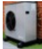
Replacement of an oil-fired boiler with a high temperature heat pump
